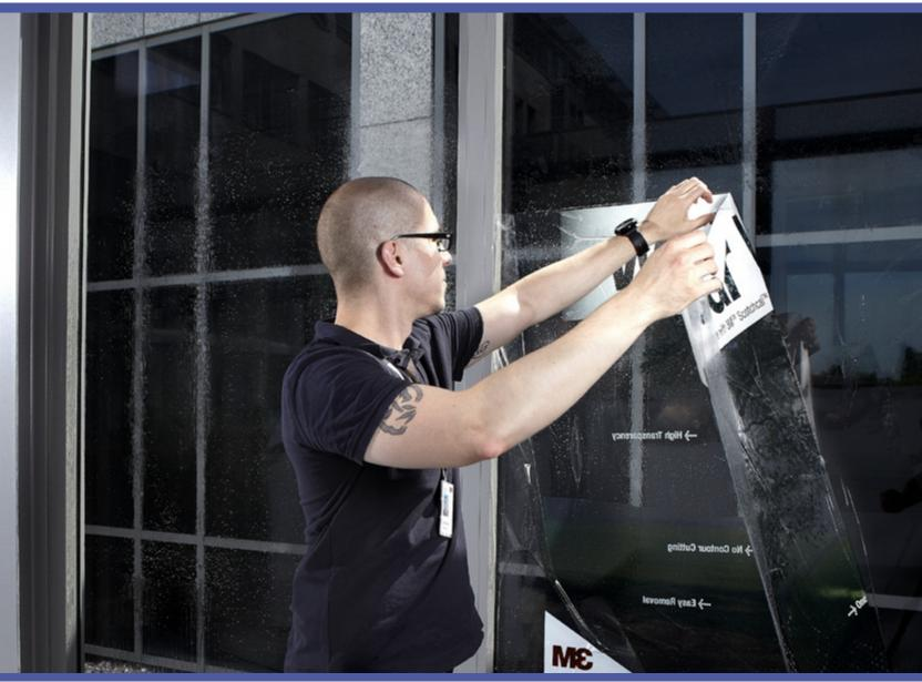
Making a perfect wet application of 3M<sup>™</sup> Scotchcal<sup>™</sup> Clear View Graphic Film 8150 | Step 10:
