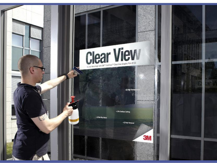
Making a perfect wet application of 3M<sup>™</sup> Scotchcal<sup>™</sup> Clear View Graphic Film 8150 | Step 15:
