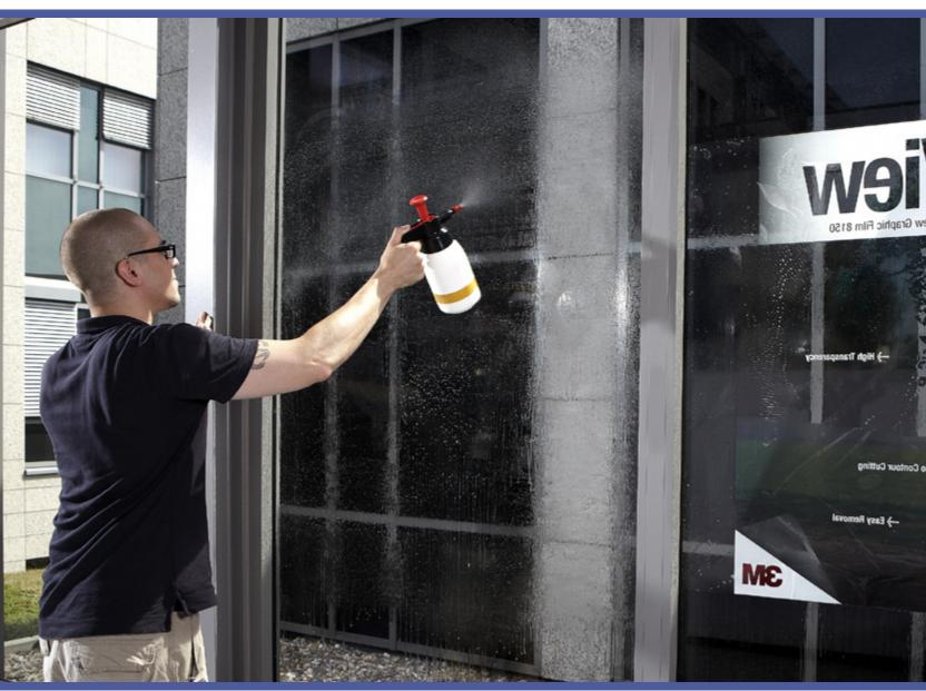
Making a perfect wet application of 3M<sup>™</sup> Scotchcal<sup>™</sup> Clear View Graphic Film 8150 | Step 9:
