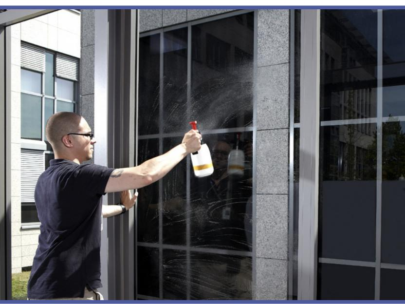
Making a perfect wet application of 3M<sup>™</sup> Scotchcal<sup>™</sup> Clear View Graphic Film 8150 | Step 3:
