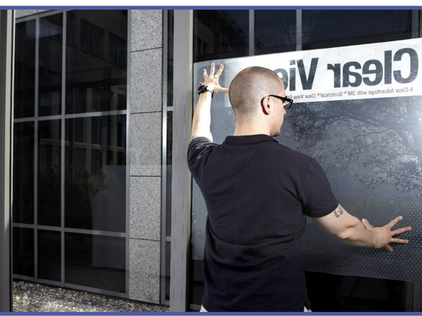
Making a perfect wet application of 3M<sup>™</sup> Scotchcal<sup>™</sup> Clear View Graphic Film 8150 | Step 6:
