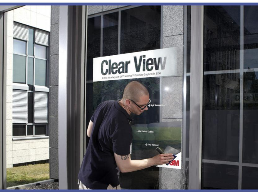
Making a perfect wet application of 3M<sup>™</sup> Scotchcal<sup>™</sup> Clear View Graphic Film 8150 | Step 17:
