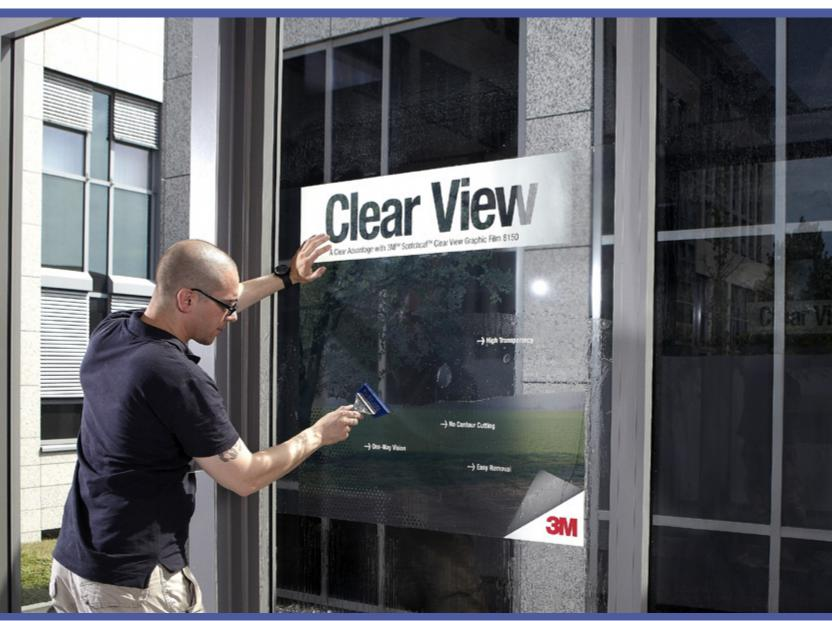
Making a perfect wet application of 3M<sup>™</sup> Scotchcal<sup>™</sup> Clear View Graphic Film 8150 | Step 16:
