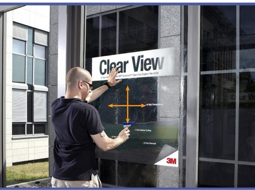
Making a perfect wet application of 3M<sup>™</sup> Scotchcal<sup>™</sup> Clear View Graphic Film 8150 | Step 14:
